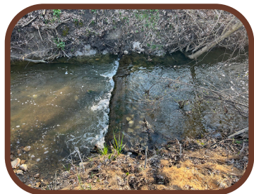
Large wood log structures were installed in the stream to stabilize the streambed and to create fish and wildlife habitat.
