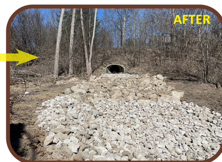
Gully filled with soil and rock riprap to keep soils from washing downstream. Invasive vegetation removed and native vegetation planted providing habitat and increased plant and animal diversity.
