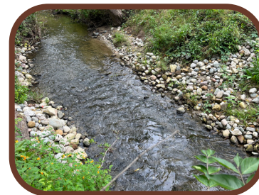
Rocks placed in stream to protect the bed and banks from erosion and provide spawning habitat for fish and other aquatic animals.
